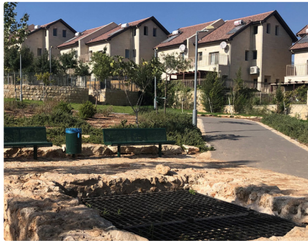
The covered shaft on the Dagan
